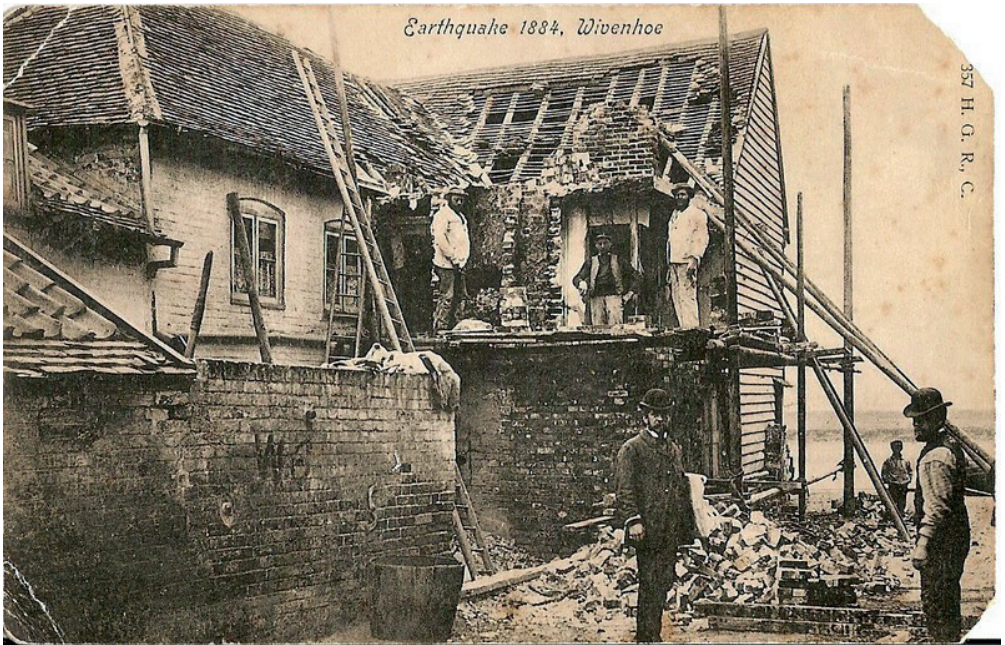
Contemporary photo postcard of damage from the 22 April 1884 Colchester earthquake at Wivenhoe, Essex.
